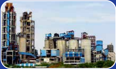
CEMENT PLANT MUKTYALA
