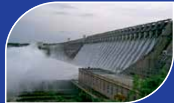
NAGARJUNA SAGAR DAM
