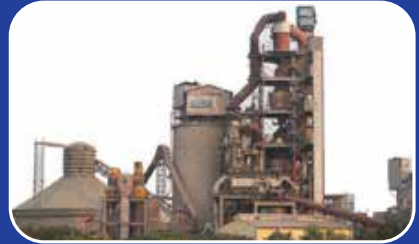
CEMENT PLANT MACHERLA
